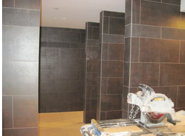
Men's Locker Room Showers
